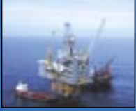
Oil and Gas Monitoring
