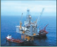
Oil and Gas Monitoring
