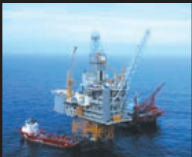
Oil and Gas Monitoring
